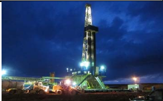
A drilling rig in North Dakota near the town of Stanley. Fracking is used in this area to tap oil reserves.
