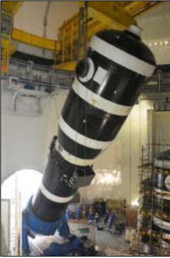
At Fangjiashan 2 a steam generator is raised to verti-
